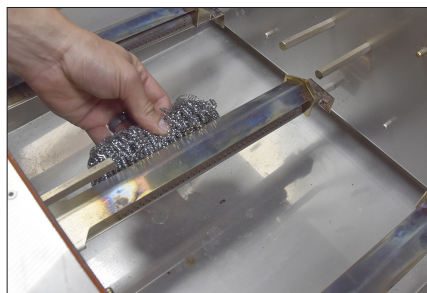
3d Cleaning debris from Burner.
